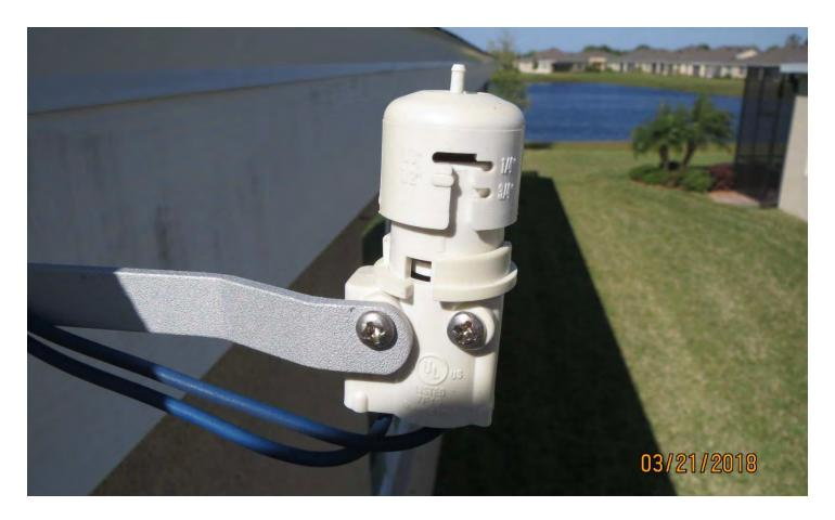
Once it was properly set, I noticed how the end of the plunger shaft sticks out of the cap at the top, so I gently pressed down and could feel a click coming from the electrical micro-switch inside the rain gauge. When this shaft is pressed down, a rain sensor icon flashed on and off in the bottom left hand corner of the control box screen, indicating the irrigation system is disabled because the cork disks are wet, swelled up, and thus pushing down on the electrical switch.
