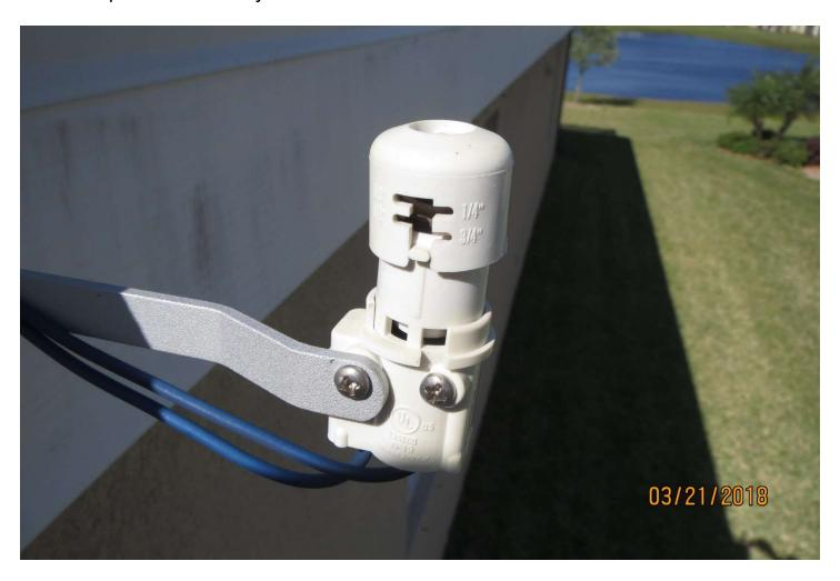
Clearly the little tab on the lower section is designed to be set into one of the 4 available slots in the cap marked 1/8", 1/4", 1/2" and 3/4" and yet there it was, not in any one of them. Being the curious person that I am, I removed the cap to see how this thing works and found a stack of cork disks on a shaft with a plunger at the bottom that presses down on the electrical switch below.
